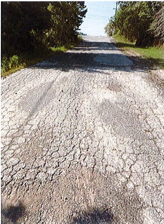
Photos 6 and 7: Pavement Distresses
